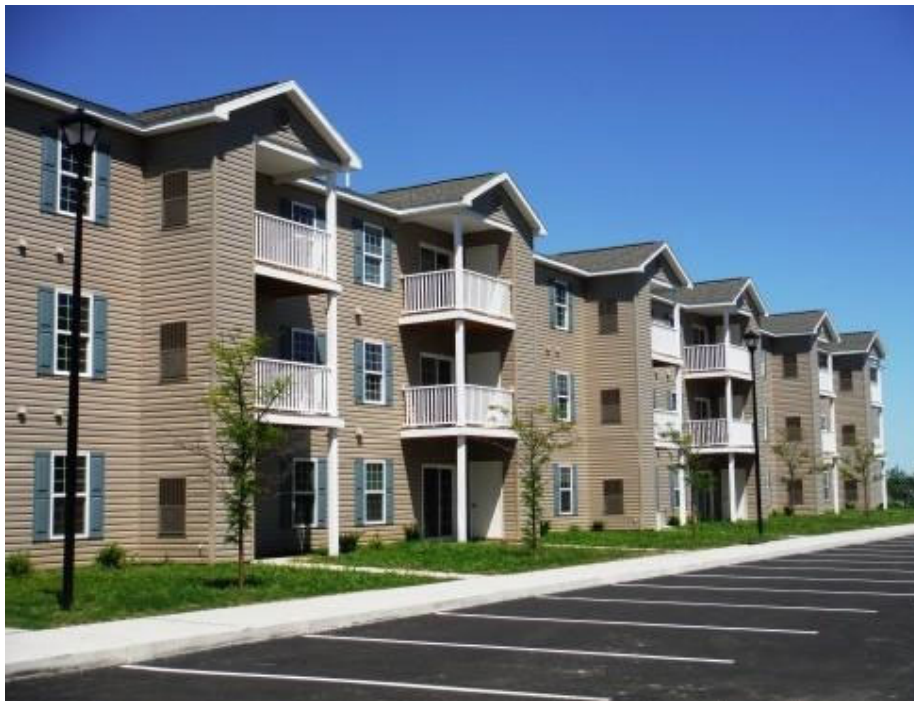
Figure B. Parking area without accessible parking or curb cuts, online photo from apartments.com of Camillus Pointe Senior Apartments, Camillus, New York.
