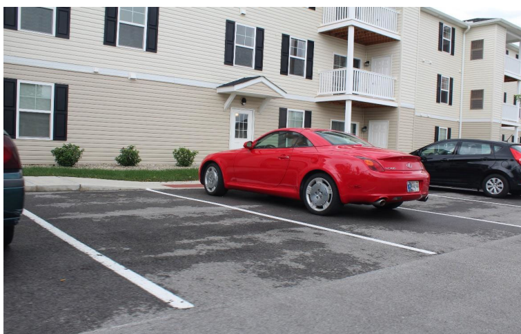
Figure C. Car blocking curb cut with no access aisle at Pleasant Run Senior Apartments, Indianapolis, Indiana.
